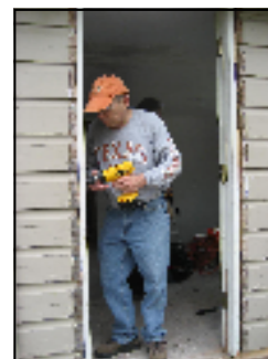
A volunteer works on a local resident's home.
